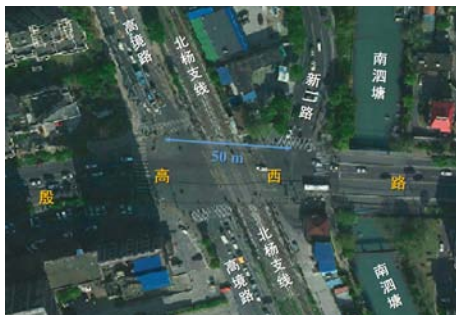
图3 殷高西路五岔路口的构成示意 Fig.3 Composition of the five-way intersection of West Yin'gao Road
