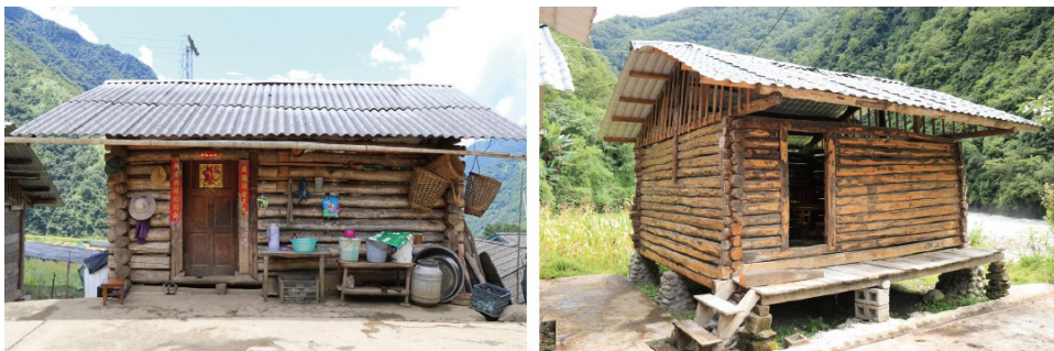
图2 独龙族传统木垒房照片 Fig.2 Photos of traditional Dulong wooden houses
