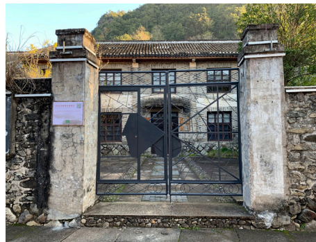
图9 改造后的电管站外观基本保持原有风貌 Fig.9 The electricity office basically maintains its original appearance after renovation
